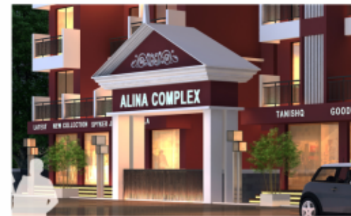
Main Entrance Gate
