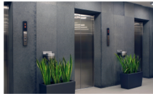
Lift with Power Backup
